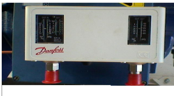
Figure : pressostat combiné HP-BP
