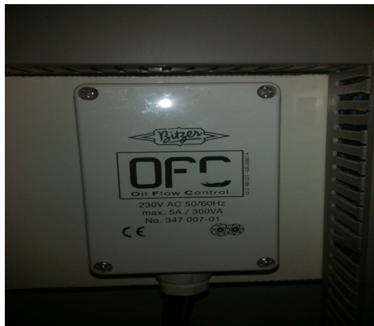
Figure : L'OFC (OIL FLOW CONTROL)
